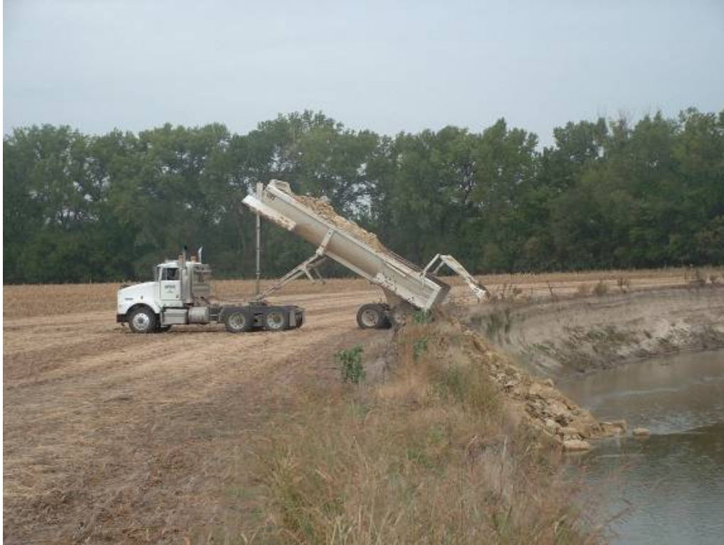
Rock weirs were constructed by the Scripters to protect from erosion a vulnerable curve on the bank of the Republican River near Morganville.
